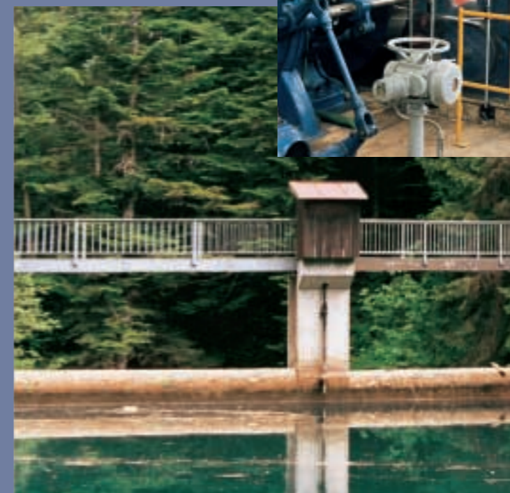
Hydro dam and turbine (at left) of the Blaichach plant, which covers approx. 60% of its electricity requirements
