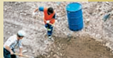
Biological soil clean-up at the Engels site ▶
